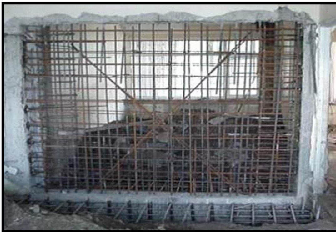
Figure 88 Addition of Shear Wall
