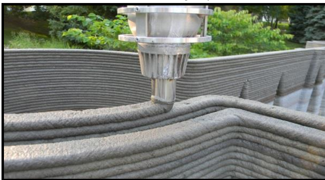
Figure 39 3D printing in construction
