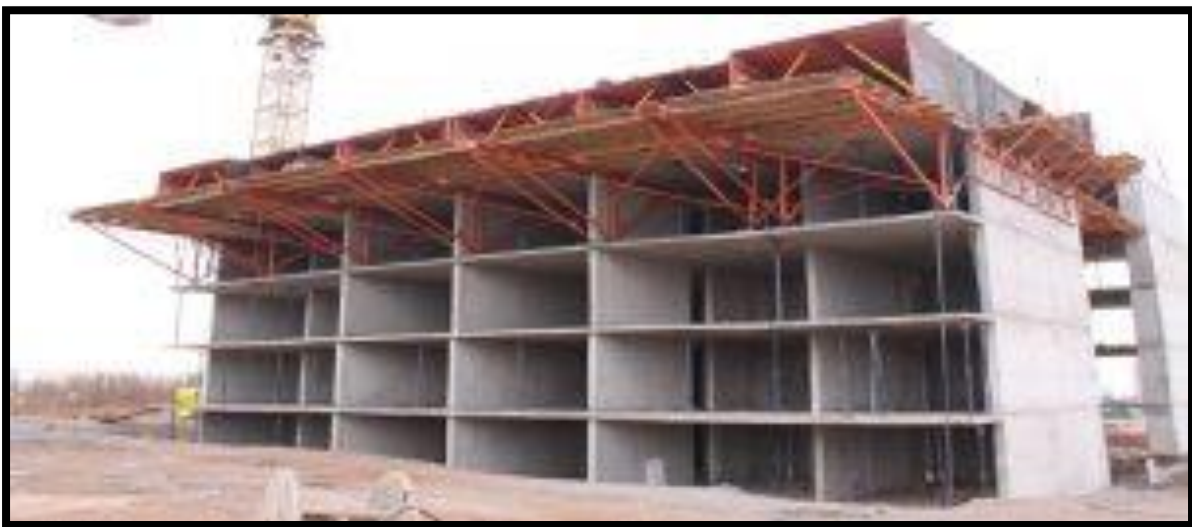
Figure 89 Tunnel Formwork System
