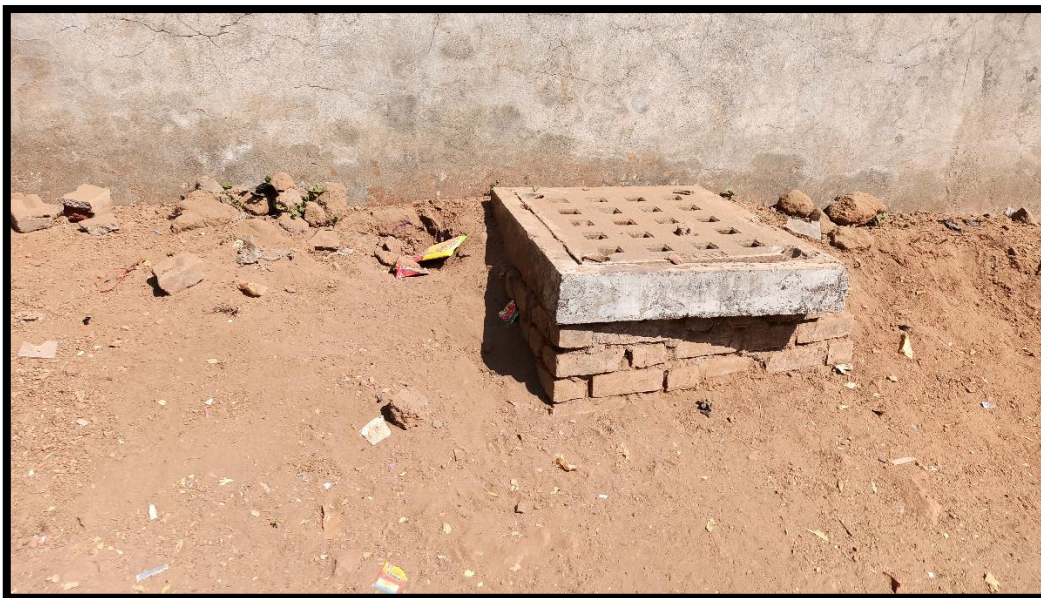
Figure 24 Manhole for underground drainage network
